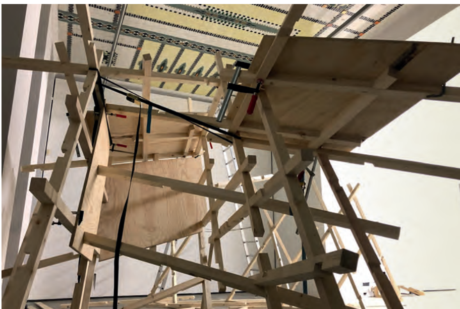
Snapshot of the Interlocking Spaces installation during the construction process, AIL Angewandte Innovation Laboratory, Oct. 2019; © conceptual joining
